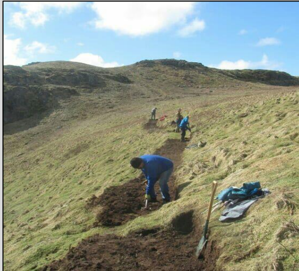
Path widening at Welsh Way in March
